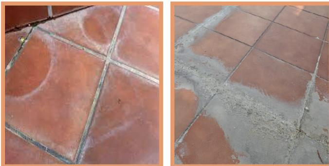
**NOTE** that Revestech waterproofing system is completely watertight and non-porous. For this reason, it is of utmost importance to follow the recommended steps to lay and install the finished flooring correctly and prevent such phenomenon as efflorescence.
