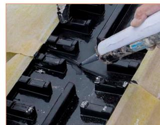
ÉTANCHÉITÉ ABSOLUE DES JOINTS GRÂCE AU SCELLÉ DE L'ADHESIF REVESTTECHFLEX.
