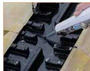
TOTAL ESTANQUIDADE DAS JUNTAS MEDIANTE VEDAÇÃO COM ADESIVO REVESTEChflex
